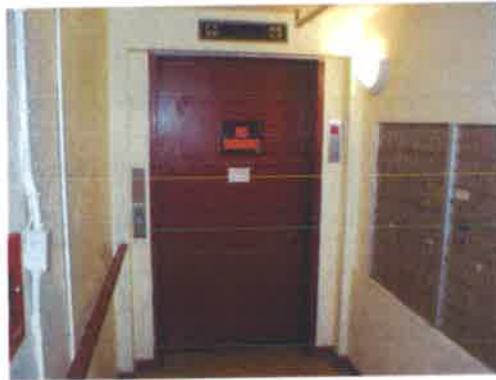
Elevator Lobby - Ground Floor
