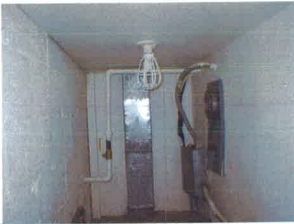
Beneath Stair Landing/Utility Closet
