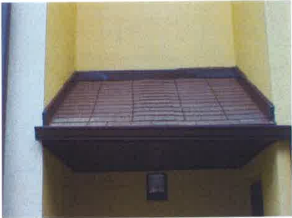
Rear Porch Roof
