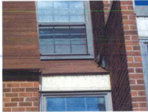
1st Floor Shed Roof
